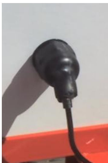
Figure 19 Sealed cable gland with heat shrink
