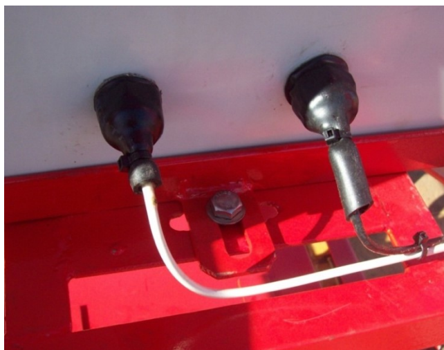
Figure 18 Sealing of antenna and power supply inputs.
